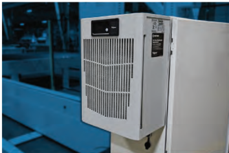
AIR-CONDITIONED MAIN CONTROL PANEL
